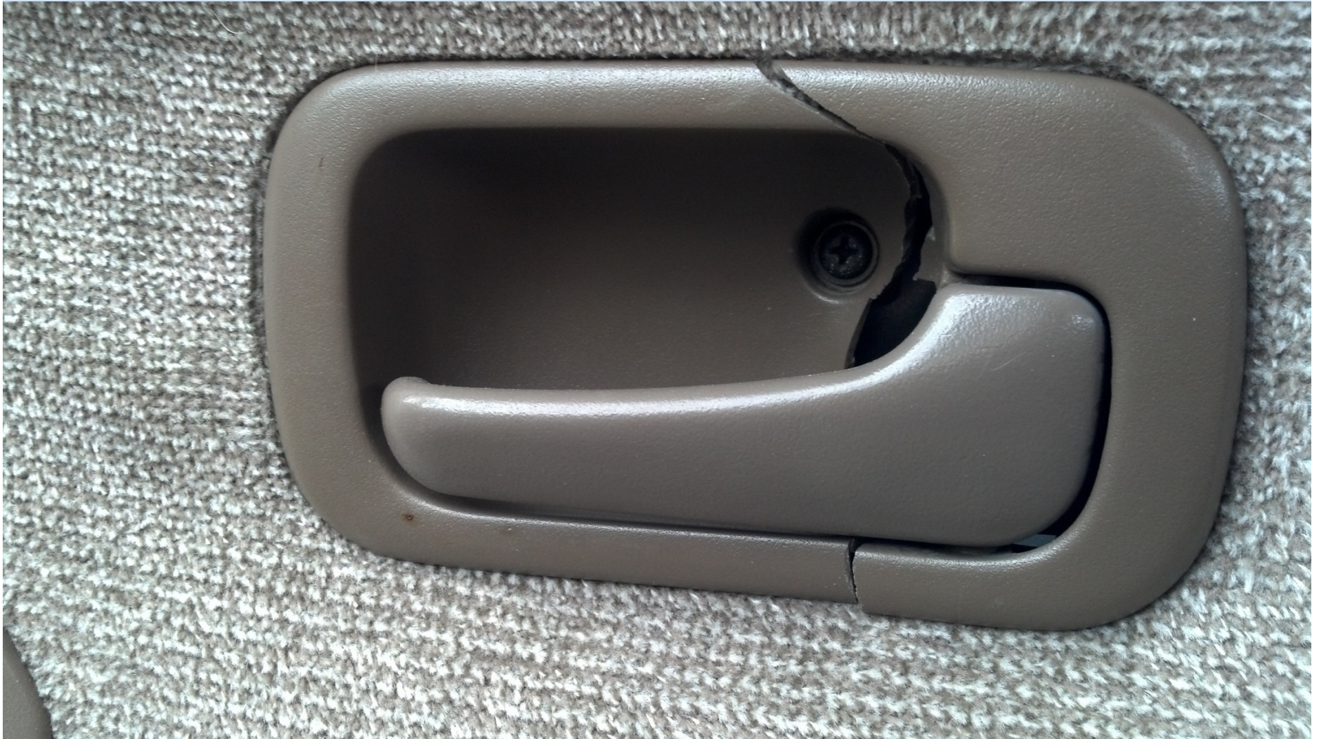
Car door handle. Cracks formed near corners rounded with a quarter circle.
